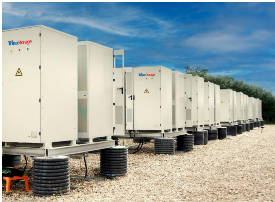
Figure 4.4.1. Close-up of BESS containers (illustration by: Kristīne Eglīte)
