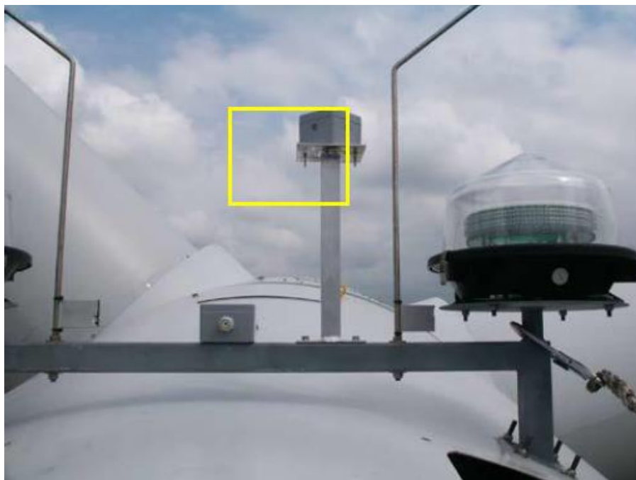
Figure 7.3.6. A light sensor is installed above the WPP nacelle to prevent shadow flicker (source: Environmental Impact Assessment of the Construction of Wind Power Plants in Tārgale Parish, Ventspils Municipality, Ltd Vides eksperti, 2022)
