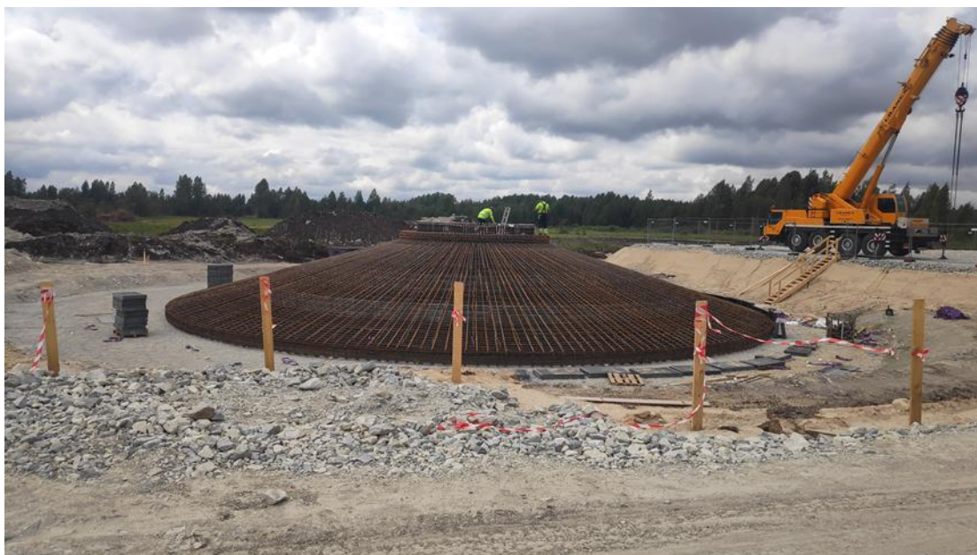
Figure 4.3.8. Part of the WPP foundation steelwork under construction (photo: Ltd Enviroprojekts)
