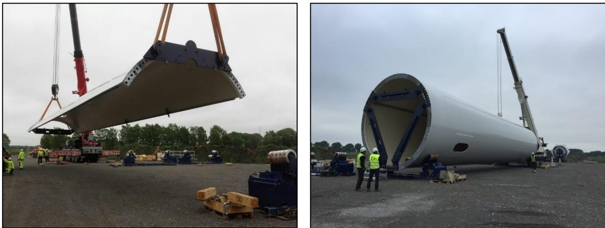
Figure 4.2.1. Multi-segment WPP mast (Vestas LDST 28 )
