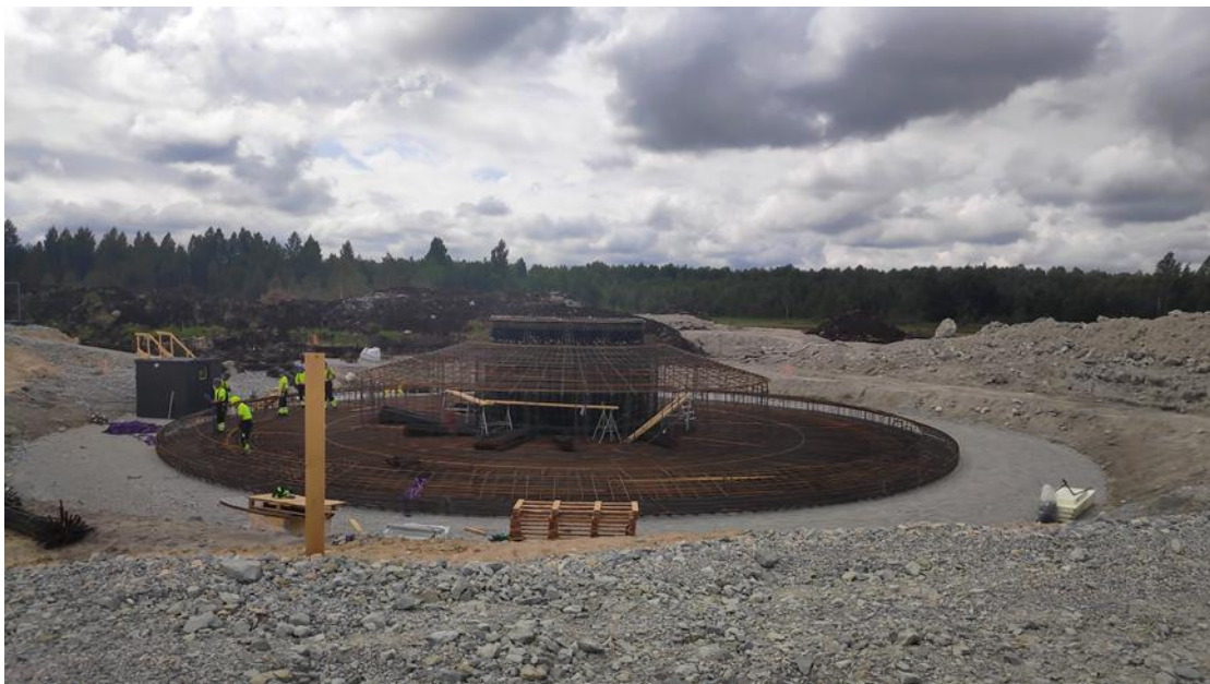
Figure 4.3.7. Part of the WPP foundation steelwork under construction (photo: Ltd Enviropojekts)
